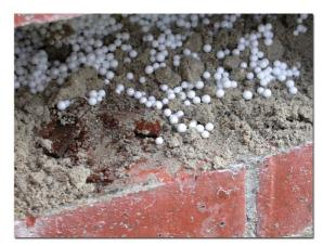
under filled, where it has slumped, where areas have been missed, vents have been blocked or obstructions missed. This is because even though the energy savings won't be as advertised there is no obvious sign of any defect. Those that are aware of a problem with the insulation within the walls will almost certainly have been put on notice with the appearance of dampness within their home.
