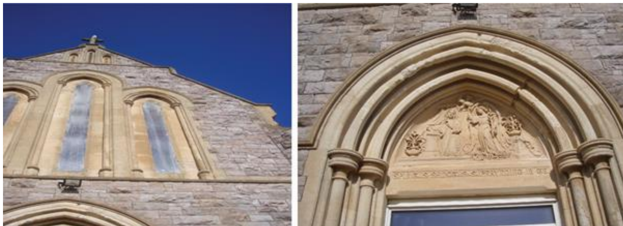
Figure 1. Holy Ghost church (Exmouth) built in 1912. Bath stone (a Jurassic oolitic limestone from SW England) was used surrounding windows and it is suffering very rapid decay. It is known that this English limestone, is not resistant to salt weathering. Its pore properties allow more moisture movement to take place inside the rock, being prone therefore to faster salt migration and more rapid degradation.
