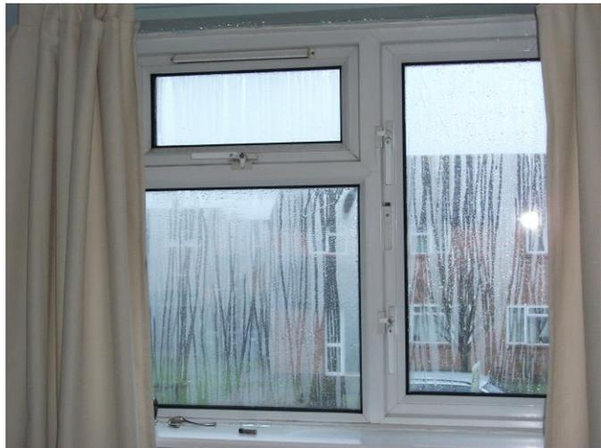
At low level, condensation may be confused with rising damp, although the moisture will usually be on the surface, superficial and hygroscopic salts will be absent. The removal of wall coverings and/or plaster will often reveal a dry substrate.
