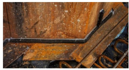
Welded sheet pile wall – floor detail with waterstop.
