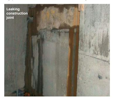
prepared to remove laitance or weak concrete as per Codes of Practice. Water stops should be used to provide enhanced resistance to water transmission at joints in the concrete structure, e.g. at construction or day work joints, services or other penetrations.
