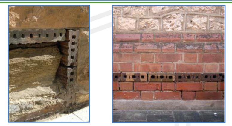
Picture: Salt attack and rising damp - A guide to salt damp in historic and older buildings
